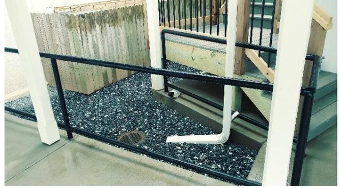
The muddy area near the new stairs and the HVAC components has been filled with gravel.
